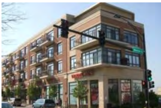
The Shops and Residences of Uptown – Park Ridge
